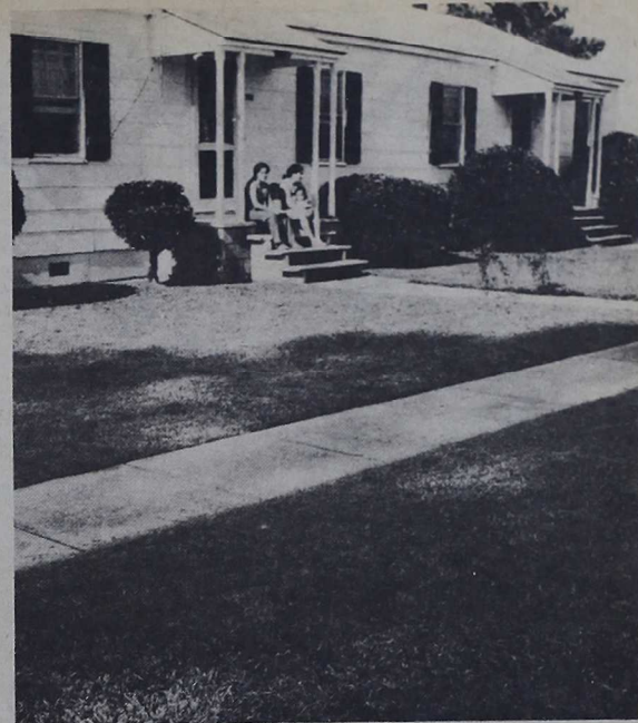
ENJOYING THE VIEW — Some Midway Park tenants visit on the front porch of their home overlooking a well-maintained lawn. A little effort in the yard makes their quarters a lot more attractive. (USMC photo by SSgt. Margarette Chavez)
