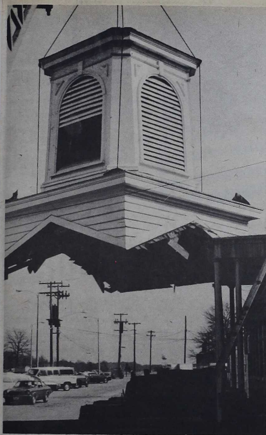
END OF AN ERA — This cupola constructed during World War II is one of nine being removed from atop Camp Lejeune dining facilities. The removal of the deteriorated cupolas, which served as ventilating fans and ornaments for dining facilities, is the first step in having new roofing installed on the dining facilities. The new roofs are expected to be completed in eight months. (USMC photo by SSgt. Brenda A. Lanclos)
