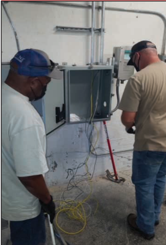
Kenneth Freeman, left and Shawn Eversole, right, both from Pine Bluff Arsenal's Directorate of Public Works, Electric Shop, work on the north side grenade line to replace Pneumatic controls and install intrinsically safe electronic controls supporting AM-14 Thermite grenades and M-330 HX grenades. U.S. ARMY PHOTO BY DPW
