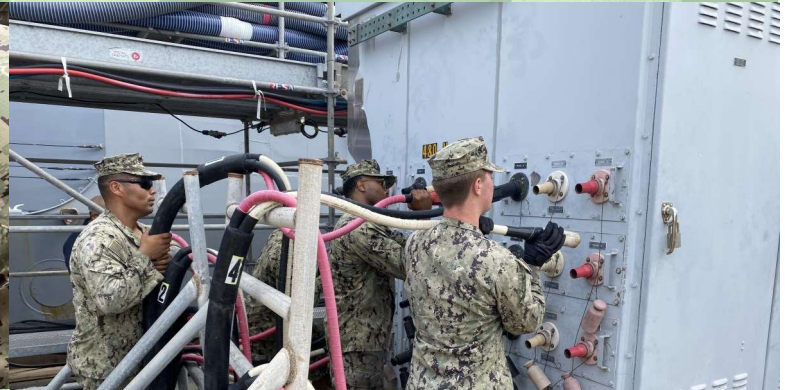
PWD Rota UEM Power Crew connect the 600-ft cable from the power mound to pier substation.
