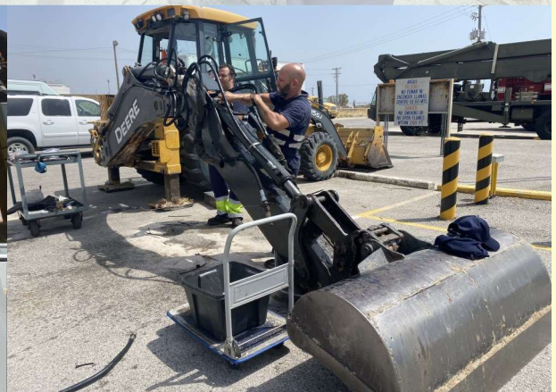
Above and Below Right: Manuel Perez Mejias and Jesus Caraballo Marquez, automotive mechanics assigned to PWD Rota Mechanics Shop, are seen here conducting repairs to a John Deere 420D Backhoe, replacing one of the hydraulic lines on the stick arm.
