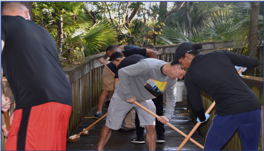
OS1 David Crider (left), AT3 Jeremiah Prendergast (center), and AT2 Gillian Mitchell (right) begin to scrub a vinegar and water solution onto a wooden bridge in an effort to remove algae growth.
