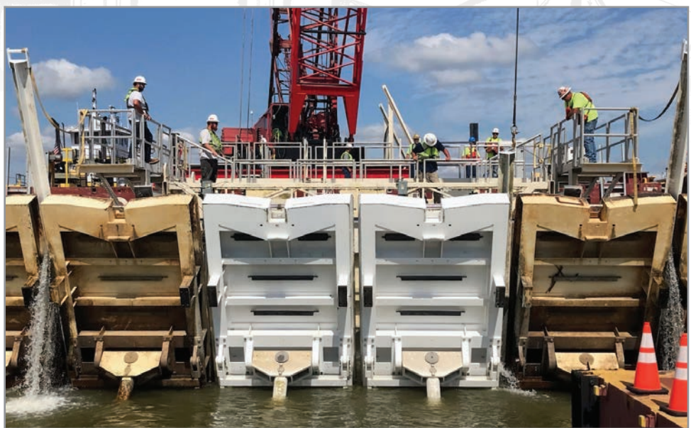
Louisville District project personnel successfully remove and replace two wickets at Olmsted Locks and Dam in Olmsted, Ill., on Sept. 14, 2021.
