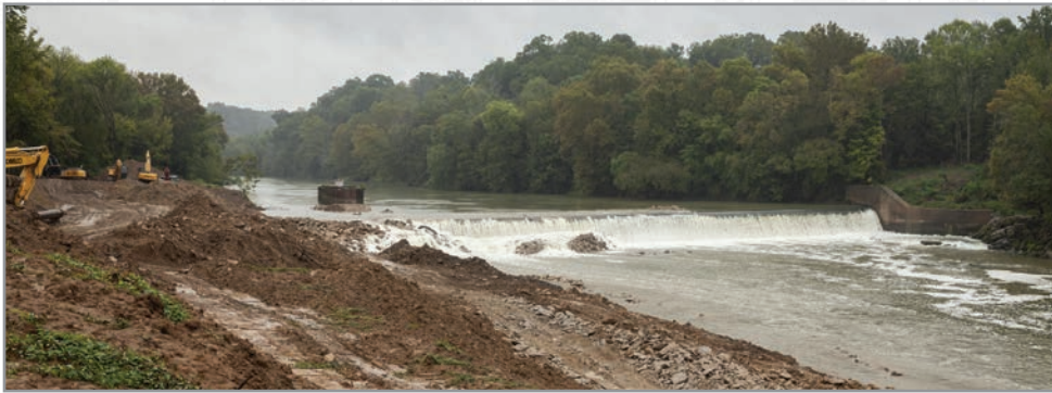
The removal of Green River Lock and Dam No. 5, near Roundhill, Ky, will restore free-flowing conditions to 73 miles of the Green River.
