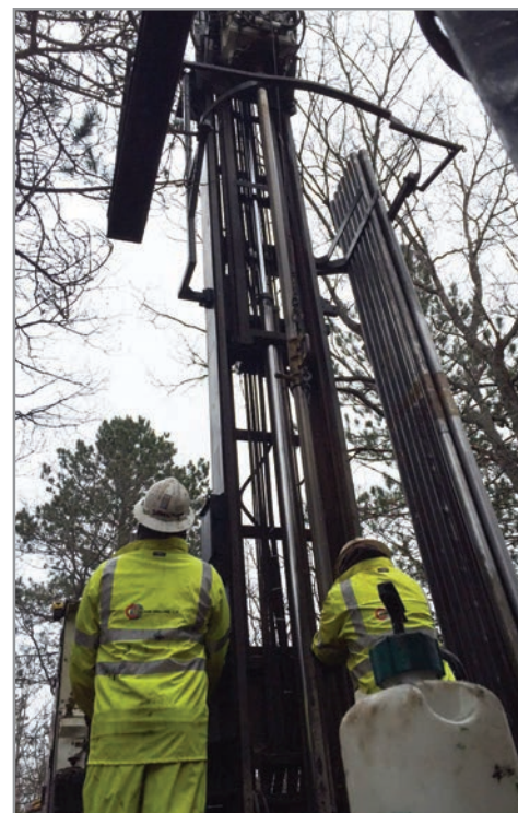
Contractors install monitoring wells at Racine Army Airfield and Missile Site in Michigan as part of the Defense Environmental Restoration Program - Formerly Used Defense Sites.
