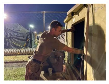
Construction Mechanic 2nd Class Joseph Bergan repairs an environment control unit (ECU) supporting the living facilities constructed for evacuees from Afghanistan at Naval Station (NAVSTA) Rota, Aug. 29, 2021. (U.S. Navy photo by Lt. Chanhan Lee)
