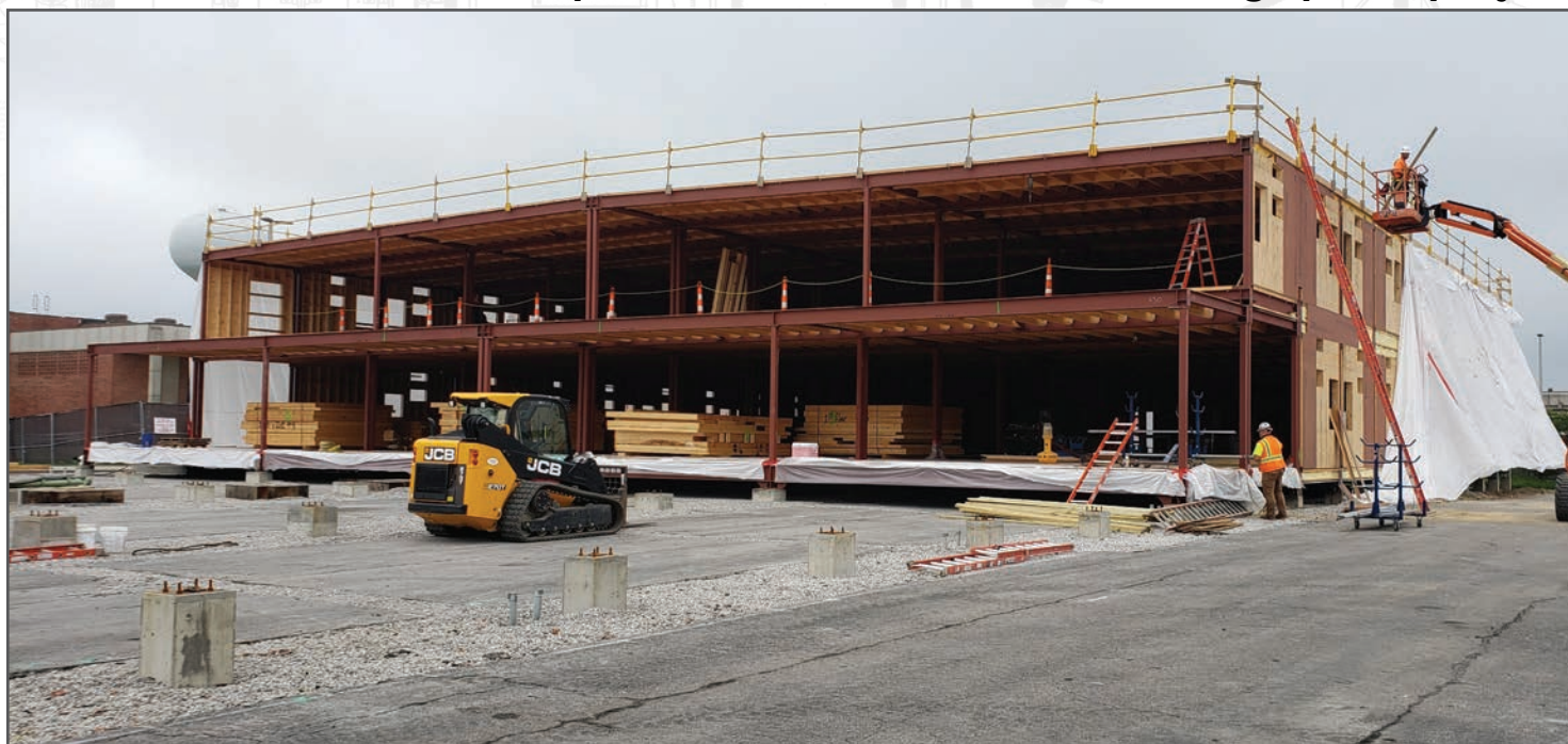
The Scott Air Force Base Air Mobility Command swing space project included the construction of a 55,000 square foot, two-story, steel-frame office building intended to house 450 personnel. The project finished on time with less than 0.5 percent modifications.
