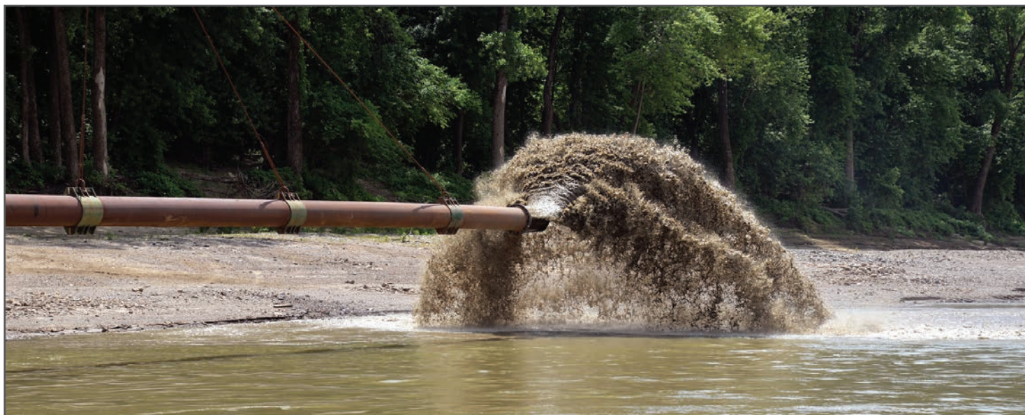
The Louisville District dredges approximately a million cubic yards of silt and sediment from more than 10 sites along the Ohio River each year to ensure safe navigation for the towing industry.
