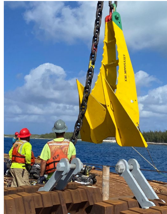
Crane lift of the new Vryhof Stevshark Rex anchor on its way to the sea floor.
