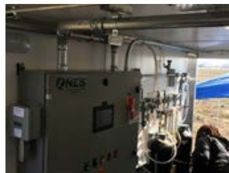
Figure B: Pilot-scale scorpion unit processes used to treat PFAS-impacted groundwater at an undisclosed Navy site – NAVFAC Headquarters funded project. (Courtesy U.S. Navy Photo)
