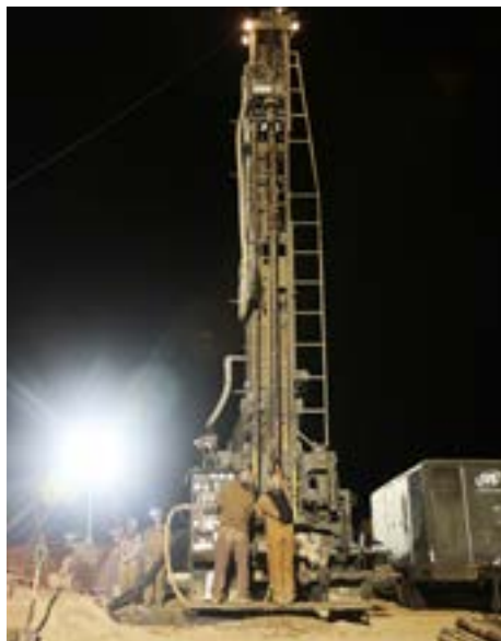
U.S. Navy construction mechanics work on the Columbia water well during drilling operations in Riohacha, Colombia. Right and left photo credit: Petty Officer 1st Class Grant Ammon
