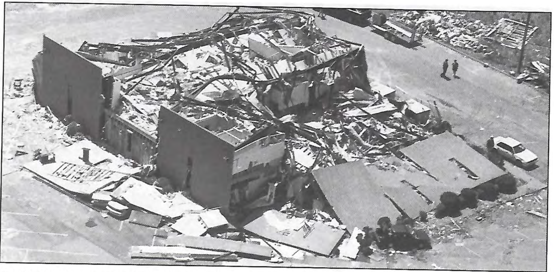
Nearly 70 people were attending Wednesday night worship services at the Open Door Church when the tornado struck and collapsed the roof. Miraculously, no one was injured even though the worshipers had to climb through windows to get out of the building.
