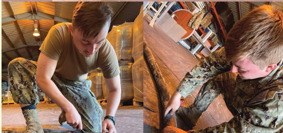
CECN Ethan Edwards (Left) and CECN Riley Novotny (Right) are seen here cutting installation on shore power cables in order to create pigtails for USS Arleigh Burke.
