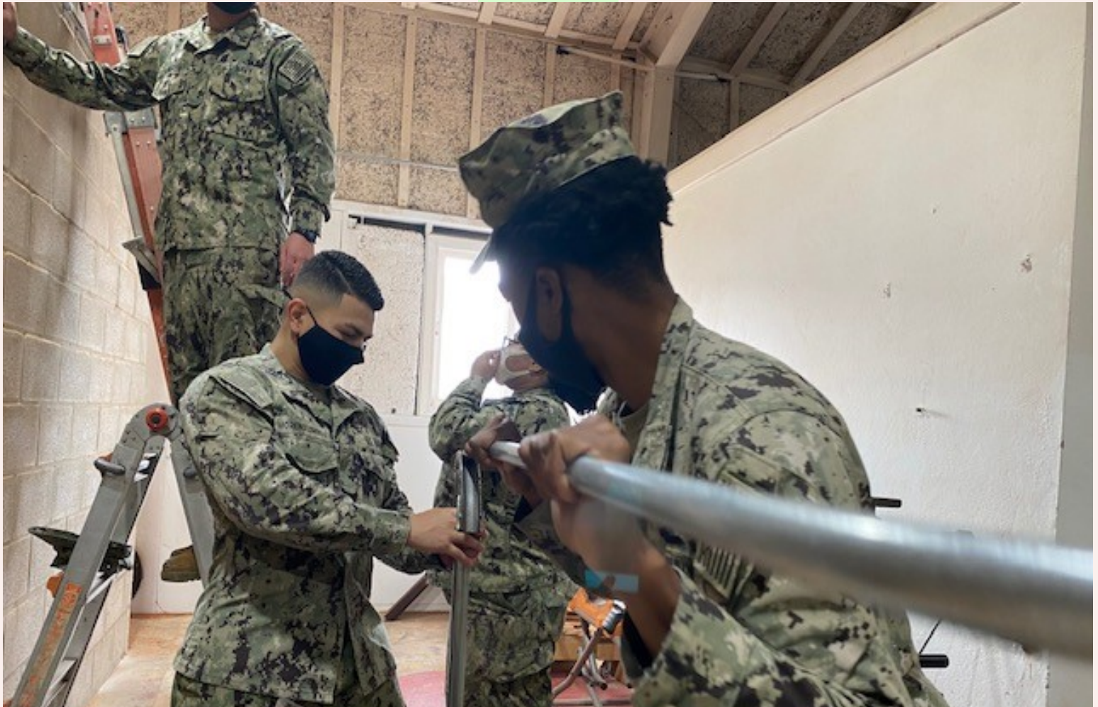
CE2(SCW/EXW) Joseph Kennedy helps CE3 Daniel Moreno bend an electrical conduit while CE2(SCW) Kiana Terry helps CECN Ethan Edwards finalize the proper measurements and height at workshop in BLDG 61. Photo and article by CE3 Daniel Moreno
