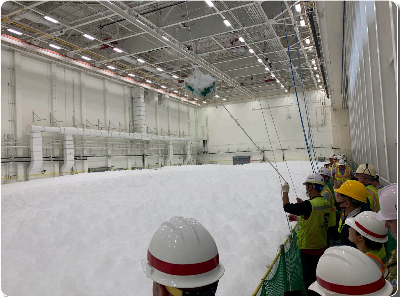
The foam is designed to cool down and seal the area involved in the fire and block oxygen, which would extinguish an anticipated jet fuel fire and halt damage to valuable equipment. After the test, the foam dissipates within 24 hours, then the foam is cleaned by a floor-cleaning machine, collected into a storage tank, transferred into a vacuum tanker truck, and transported to a waste treatment plant for disposal. (U.S. Army photos by Sameria Zavala)
