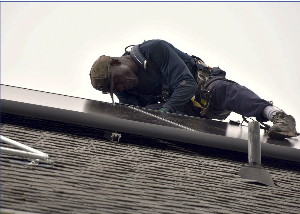
Courtesy Photo Stephen Mack with Sunrun, Inc., installs a solar panel on top of a roof in the Balfour Beatty Communities Housing Area aboard Naval Air Station Jacksonville, June 16. The project consists of placing solar panels on 185 homes to use up to 20 percent of renewable energy, reducing their carbon footprint.
