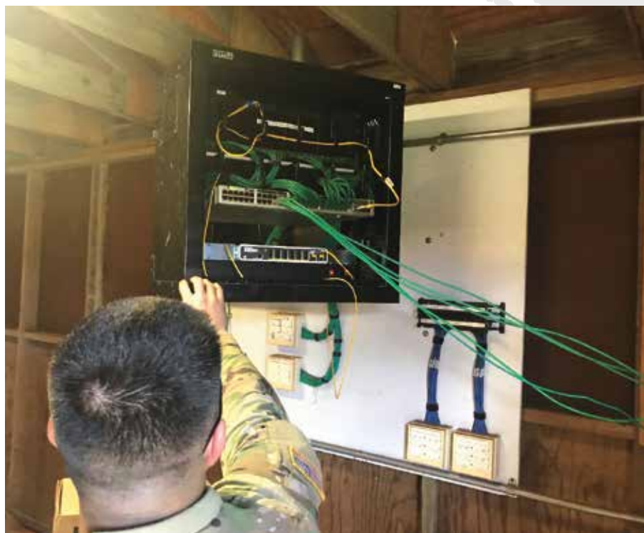
During the exercise, Soldiers configured network switches, ran fiber and Ethernet cables to all locations, and while troubleshooting information systems.
