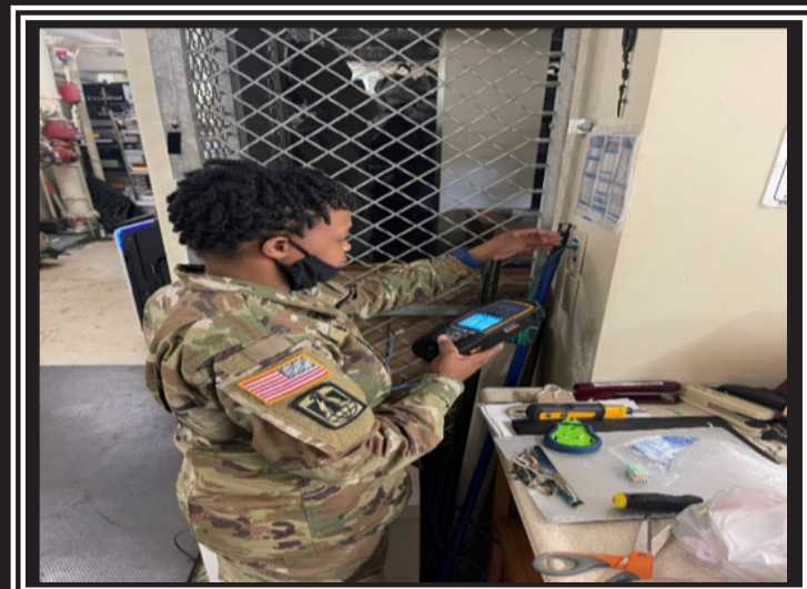
SGT Nowlin plugging one end of a Category 6 patch cable to a wall port and the other end into the Cable Analyzer in order to check proper connectivity.
