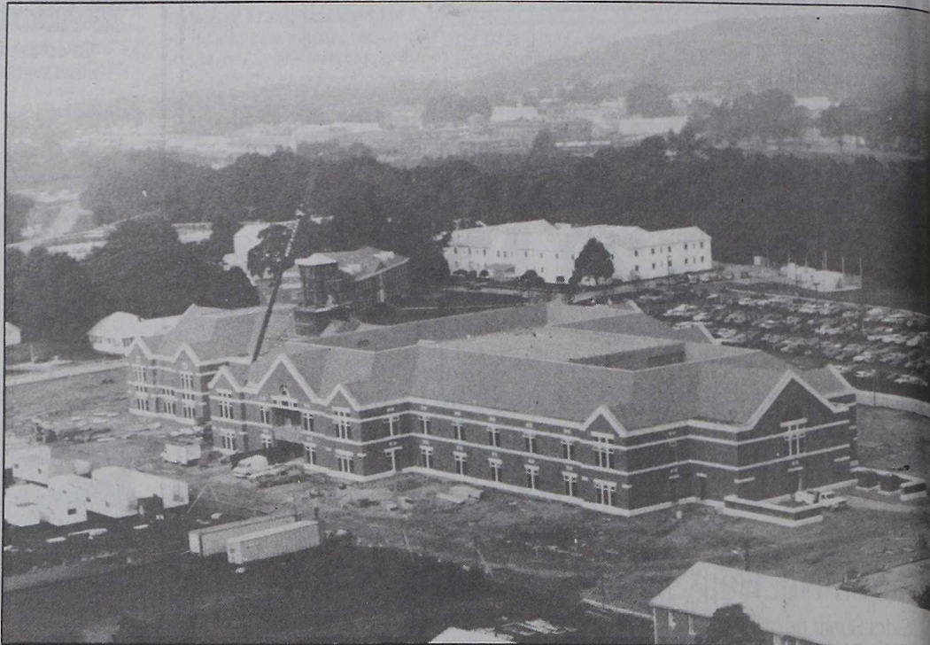
The Marine Corps Research Center under its final stage of construction as seen from an aerial view. When the center is operational, a staff of 32 personnel will perform all tasks associated with its function.
