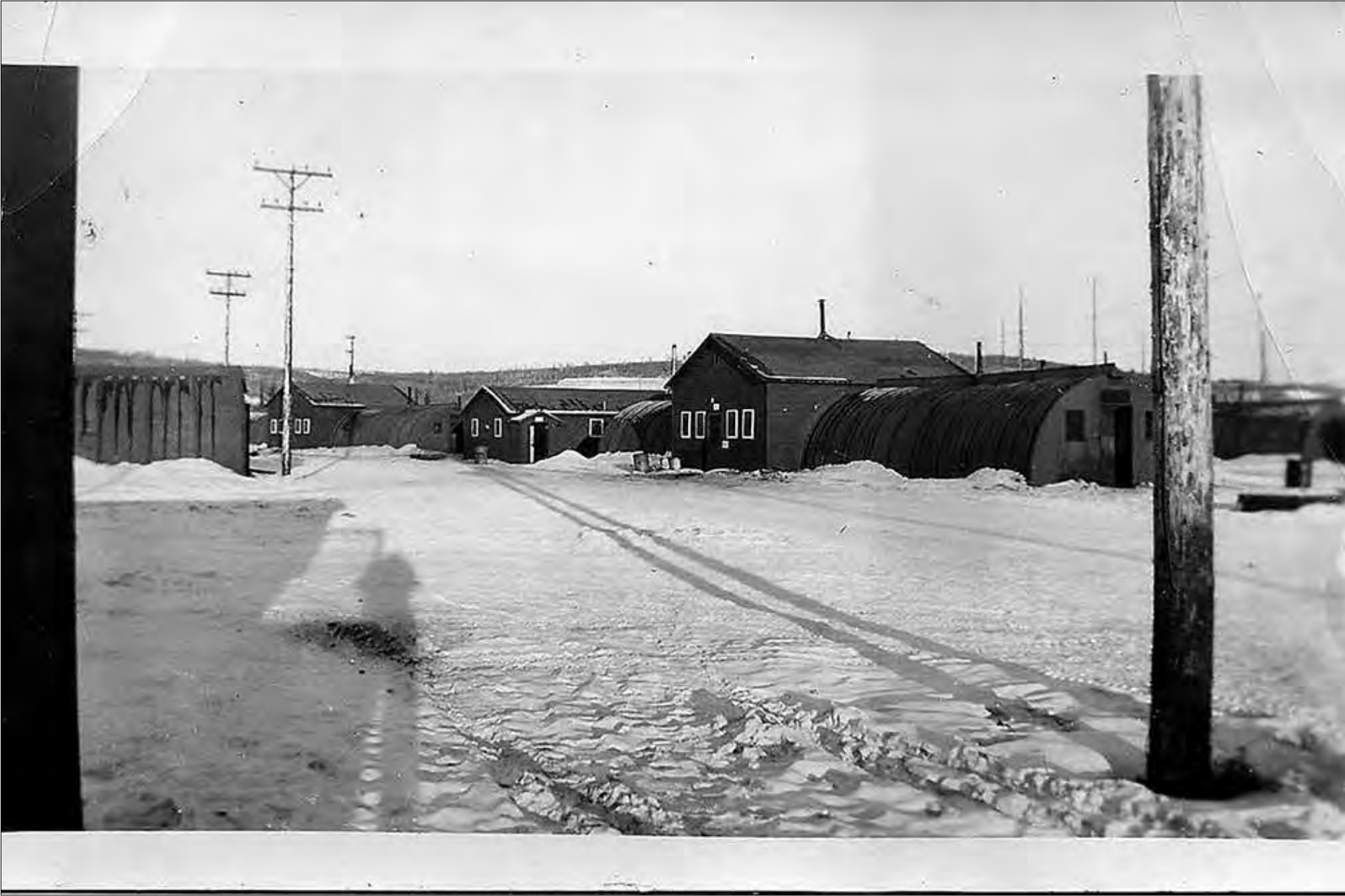
The U.S. Navy first commissioned the Quonset hut in 1941 when it needed an easily shippable, multi-use structure that could provide durable shelter in a variety of climates. Based on the British Nissan hut, the Quonset hut came in a variety of prefabricated sizes and could be assembled with no specialized training or tools on virtually any level surface, including the bare ground. Quonset huts were also easy to move once assembled and could be readily hoisted onto trucks, or even carried in one piece by a troop of strong Soldiers. At Ladd Field, hundreds of Quonset huts were hastily put up to accommodate the arrival of new Soldiers after the onset of World War II. Quonset huts were also used extensively in the Aleutian Islands. After World War II, unneeded huts were sold to the public and repurposed into schools, offices, businesses, garages, and even private homes. (Photo Harold Wright and the 46th 72nd)
