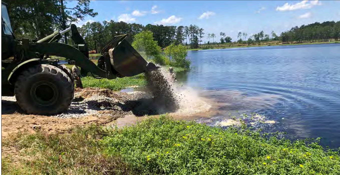
An equipment operator uses a loader to place gravel.
