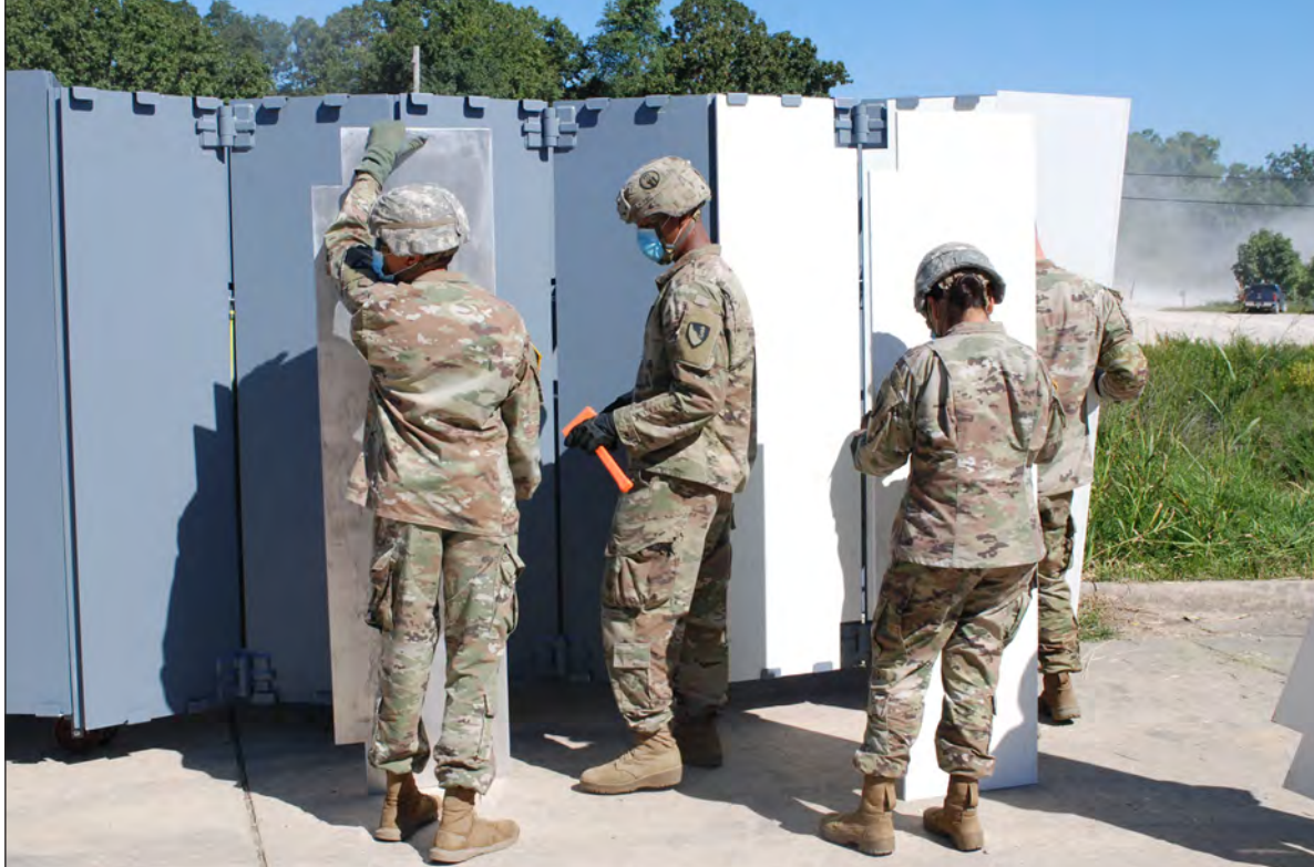
Deployment of the RAPID system with E-Glass ballistic panels installed.
