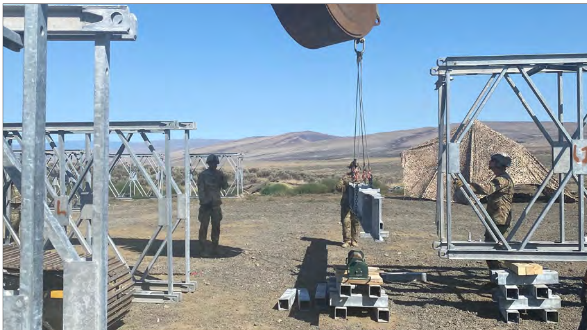
Figure 2. A transom is lifted into place.
