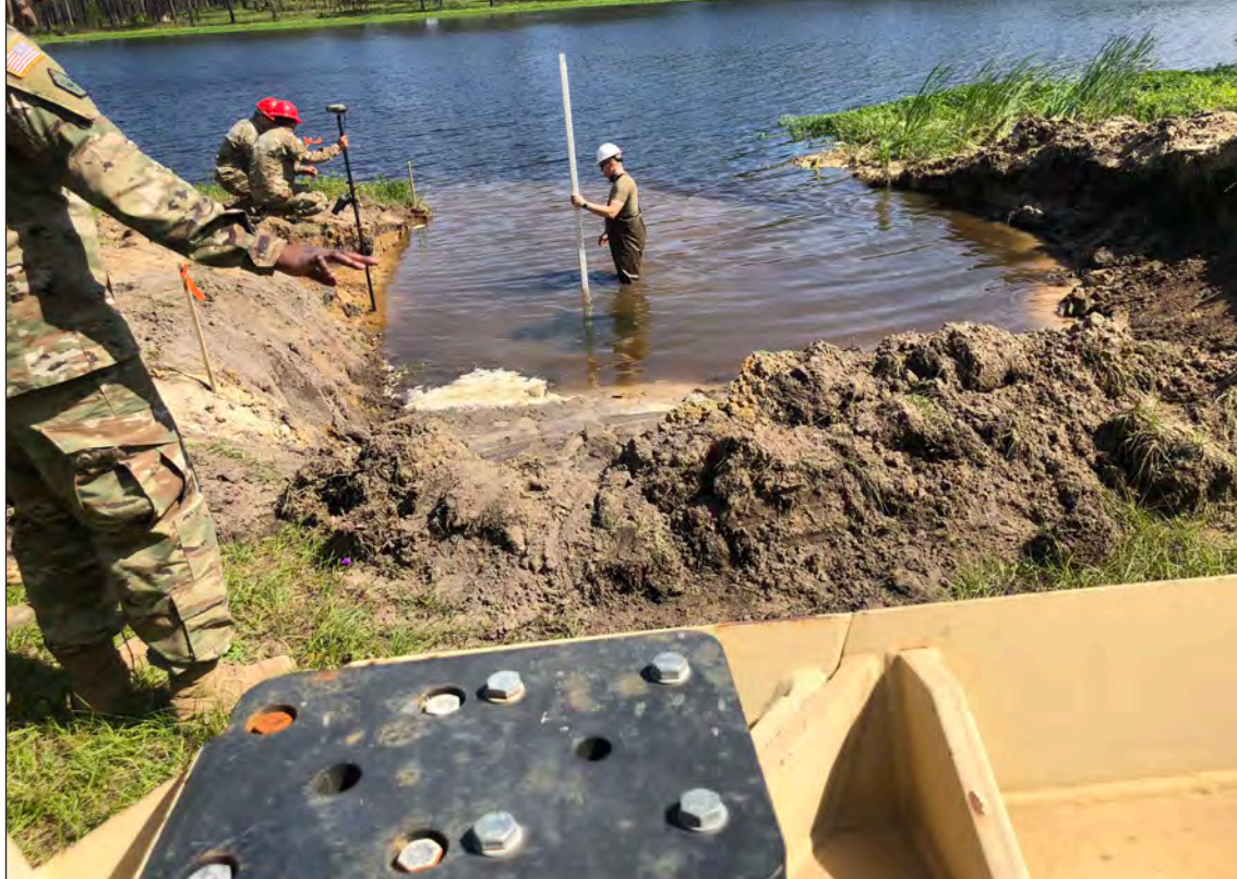
Surveyors verify water depth for a ramp.
