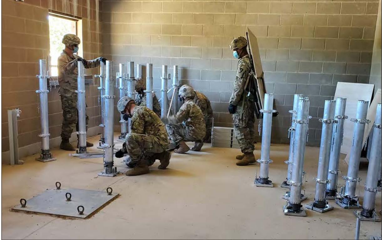
Soldiers setting up an expedient retrofit for existing buildings.
