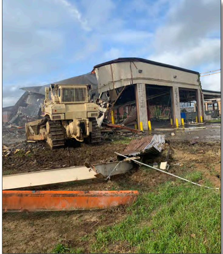
Demolition of a maintenance bay
