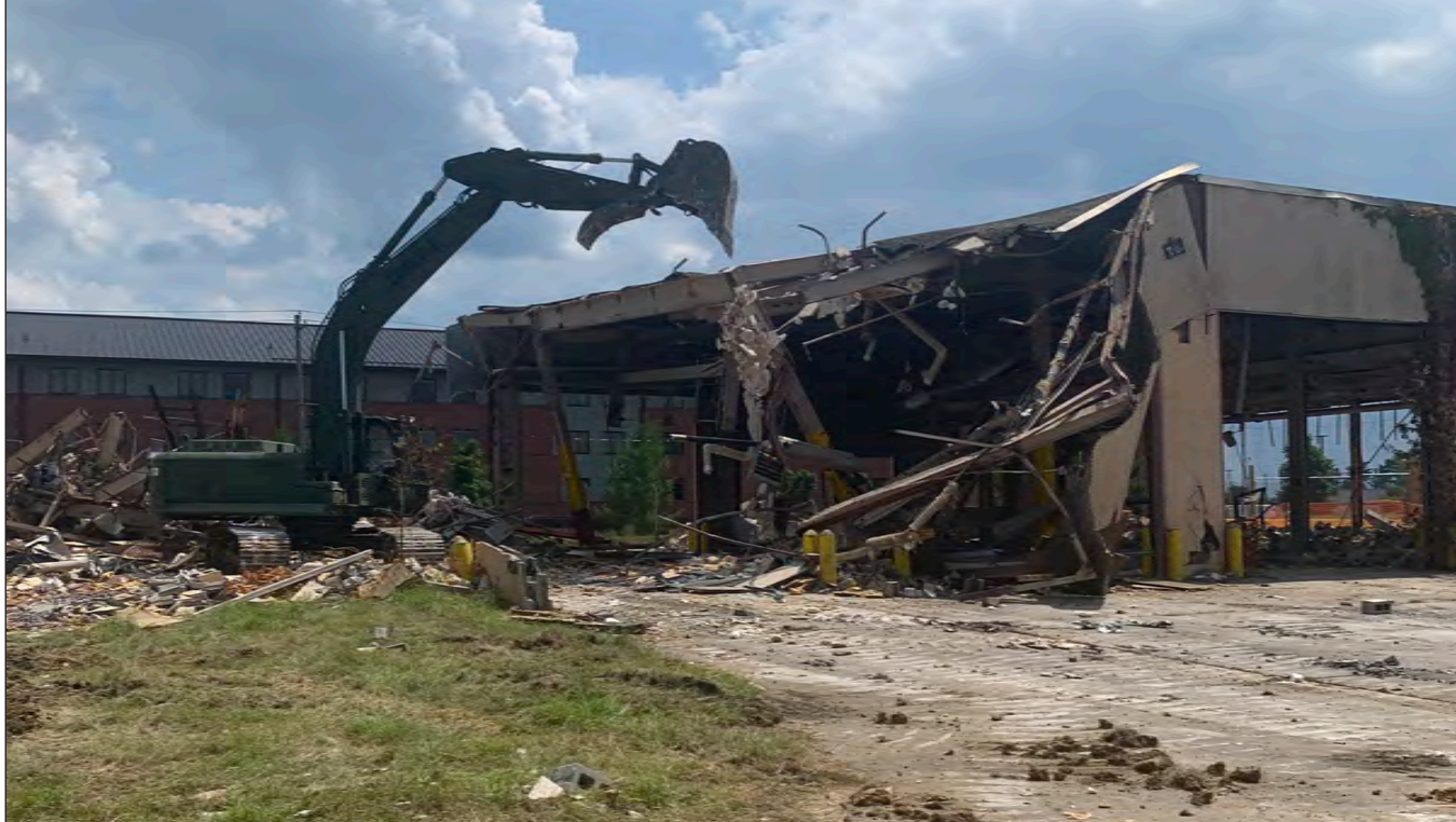
Excavator demolition on a maintenance bay
