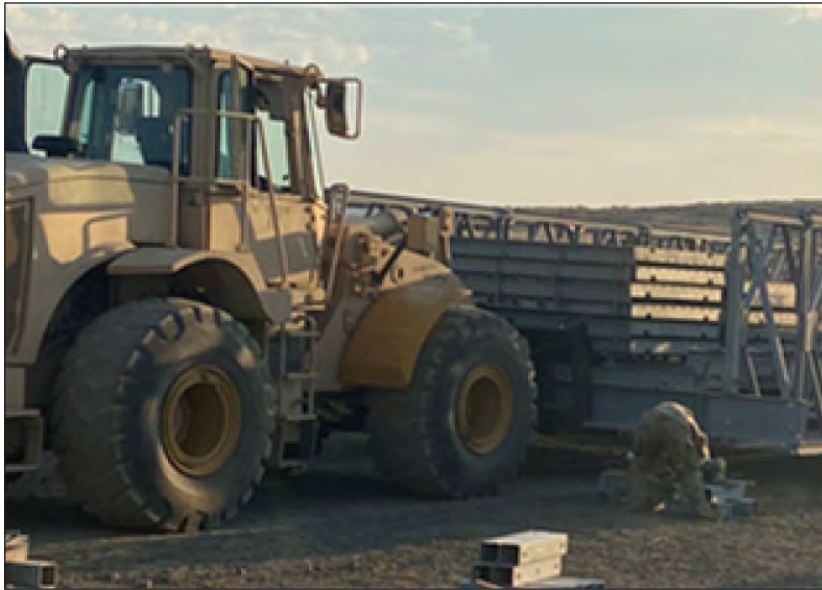
Figure 3. A forklift is used to launch the bridge across the gap.
