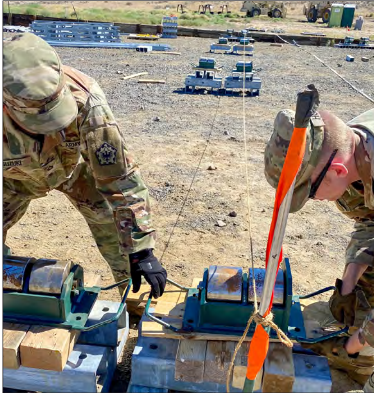
Figure 1. Soldiers placing rollers during site layout
