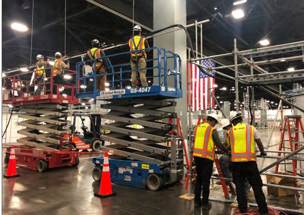
Installation of oxygen, power, and network lines at MBCC
