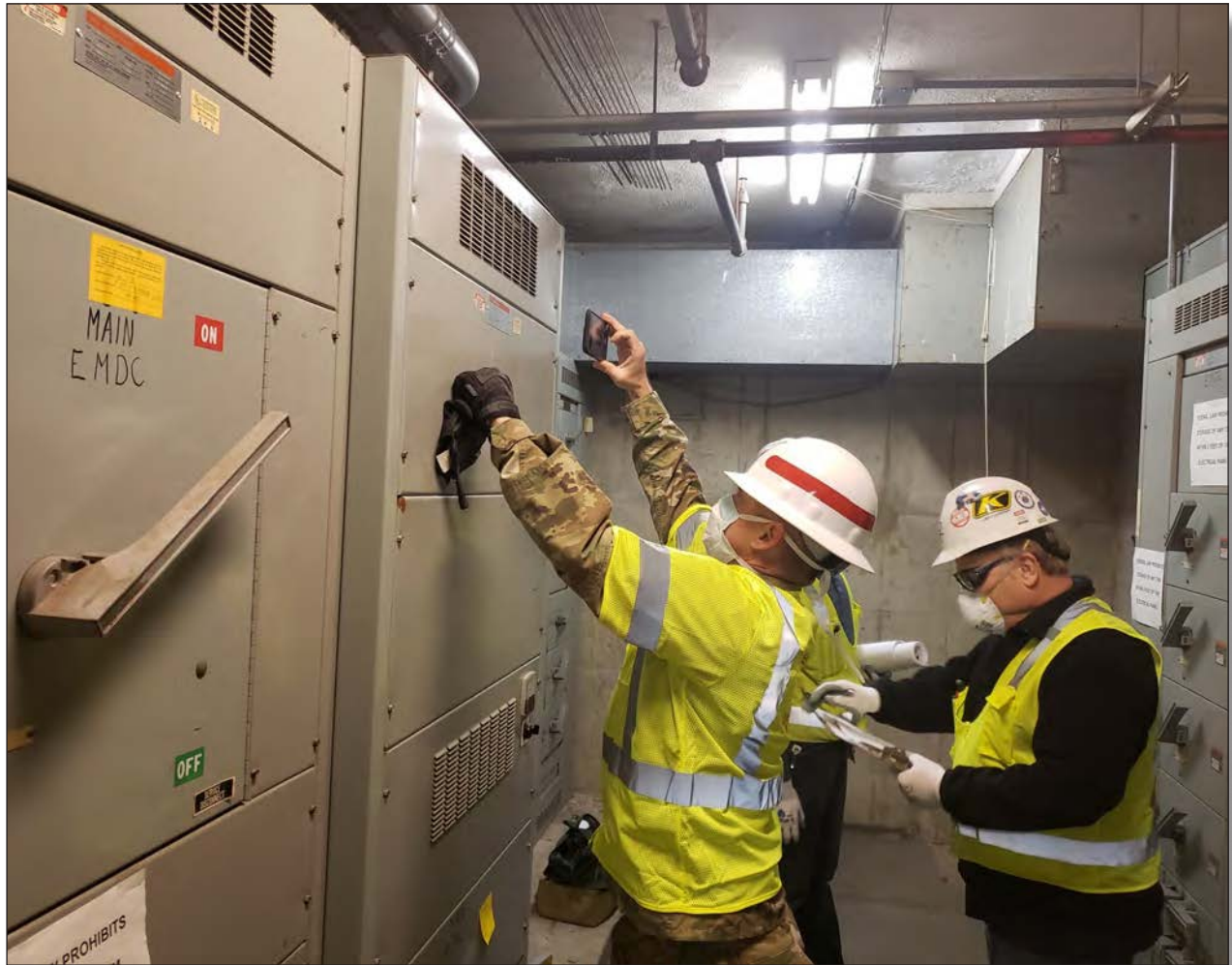
Contracting-team members conduct a power load assessment at an alternate care facility.
