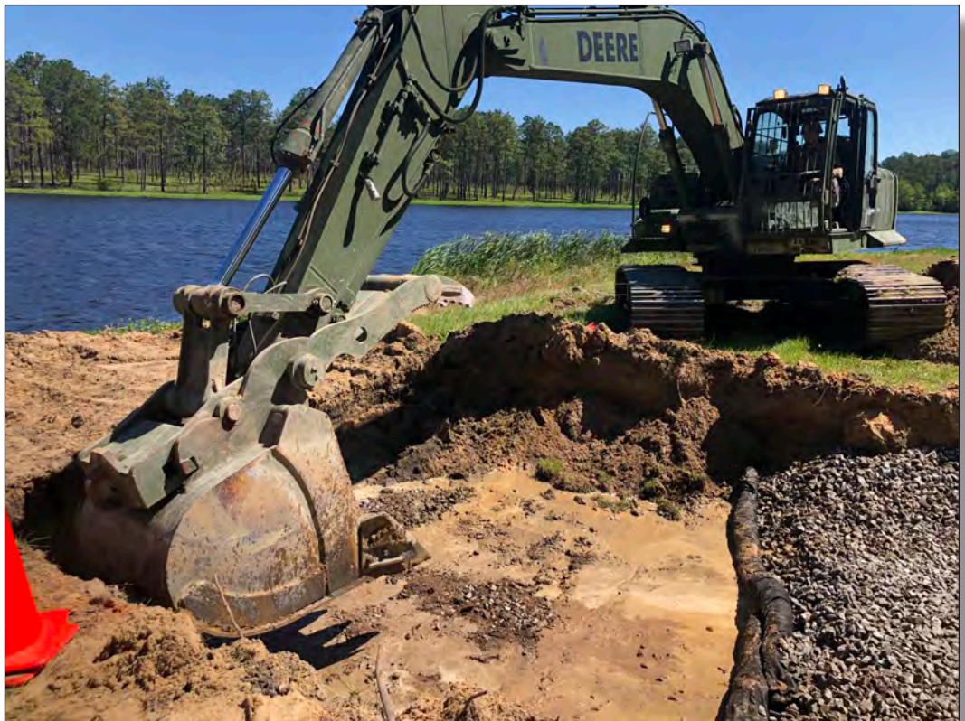
An equipment operator uses a hydraulic excavator to cut the surface for a designed slope.
