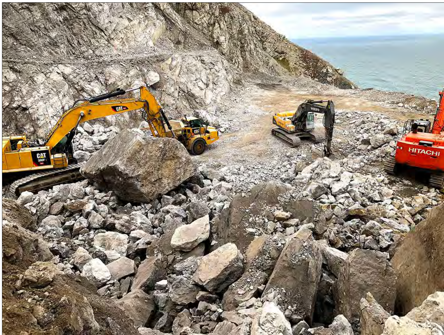
Workers excavate rocks from a quarry on property managed by the U.S. Fish and Wildlife Service near Cape Lisburne on Sep. 24, 2019. Repairs to the seawall required four different sized rocks, ranging from large boulders to small stones. Using the nearby quarry prevented the need to ship rocks from other sources and meant finishing the project at a quicker pace.
