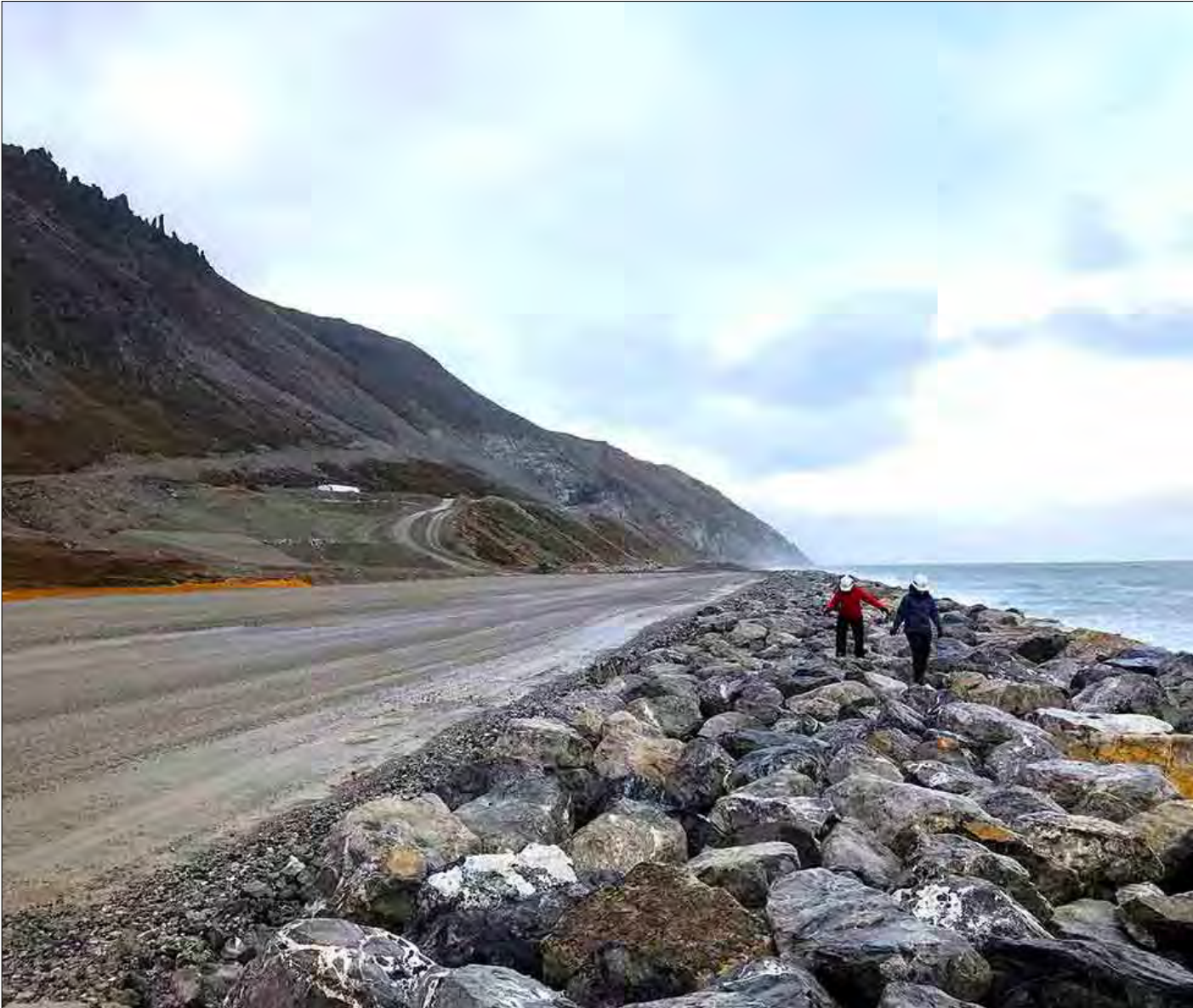
Julie Mages, deputy base civil engineer at the 611th Civil Engineer Squadron, and Lauren Oliver, hydraulic engineer at the U.S. Army Corps of Engineers – Alaska District, assess the seawall at Cape Lisburne on Sep. 30, 2019. The protective barrier prevents harsh waves and ice from flooding and damaging the adjacent runway, which serves as the primary avenue for people and supplies to reach the remote military base. The site is operated by the Pacific Air Forces Regional Support Center and provides aerospace surveillance to detect and allow for an early response to potential threats to North America.
