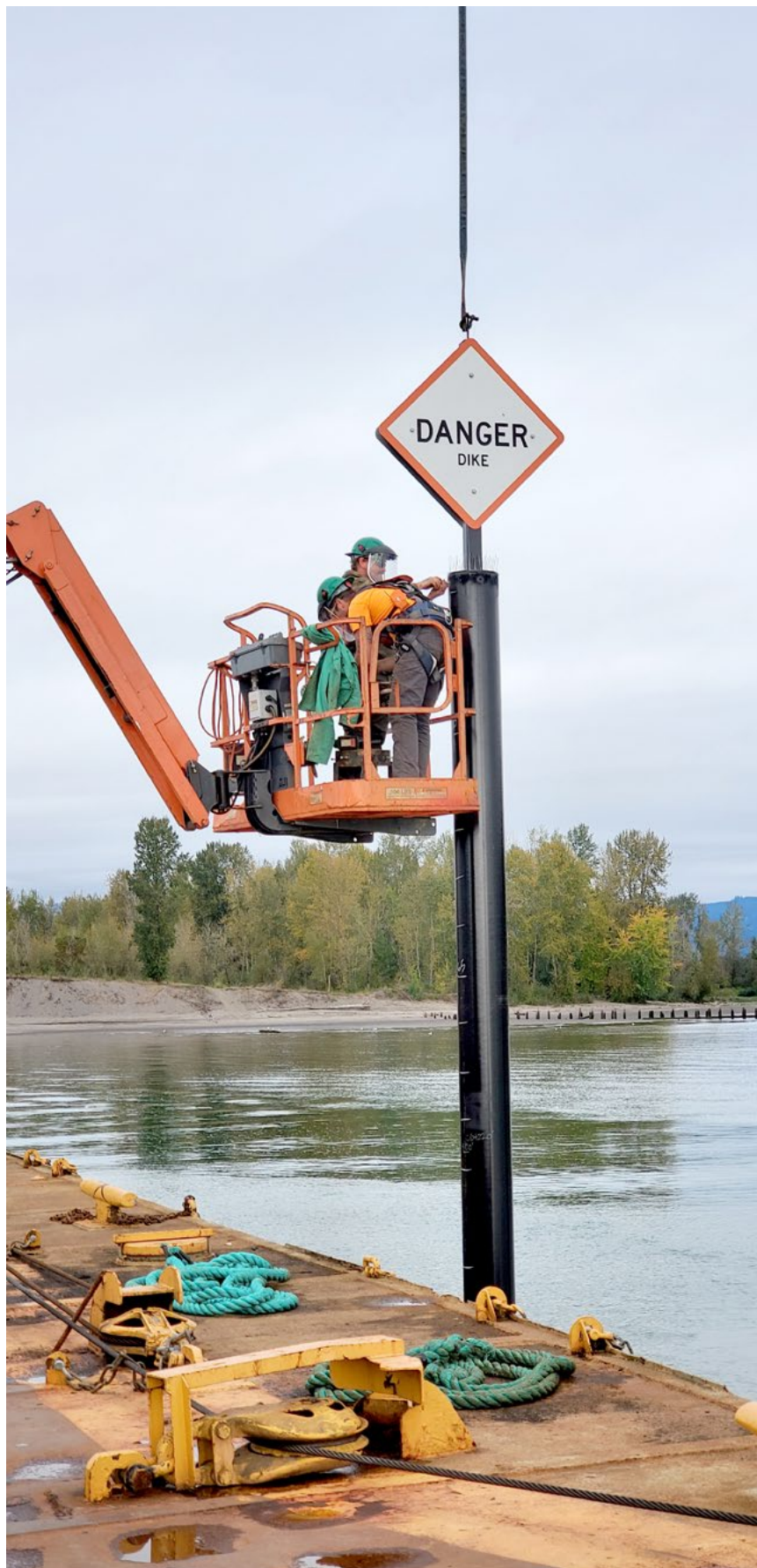
Workers installing a king pile marker warning sign.
