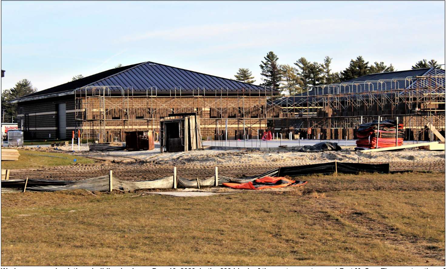
Work on a new simulations building is shown Dec. 10, 2020, in the 200 block of the cantonment area at Fort McCoy. The construction of this facility is by Contractor MDM Construction Supply of Rockford, Ill.
