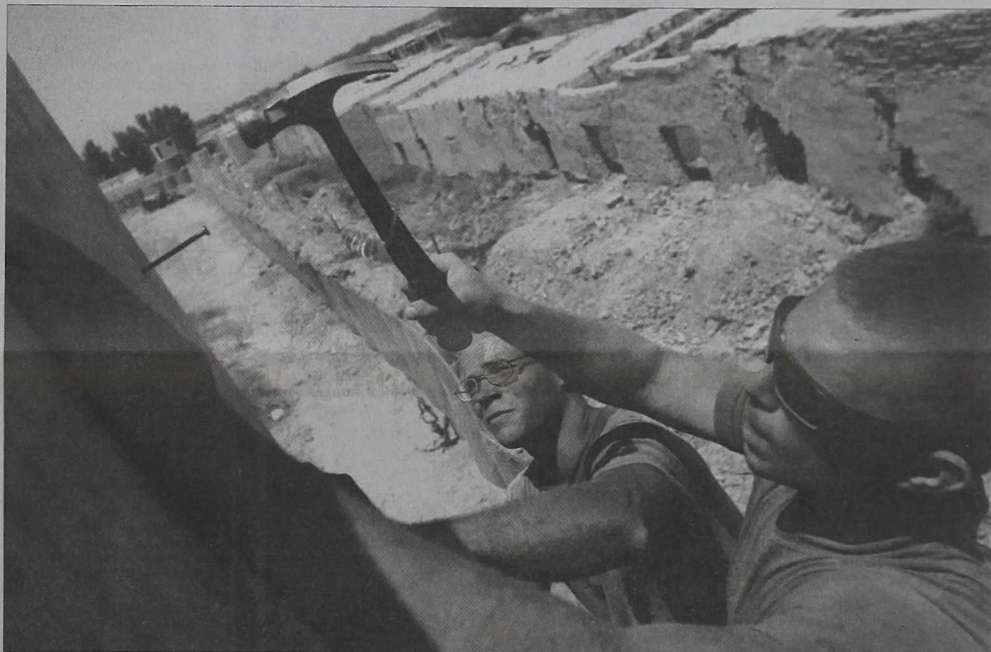
Cpl. Stephen Maloney, a combat engineer with 1st Combat Engineer Battalion, constructs an observation post at Patrol Base Jaker, July 26. Marines with 1st CEB, along with heavy equipment operators from Combat Logistics Battalion 8, have been working day and night since July 29 to expand PB Jaker.
