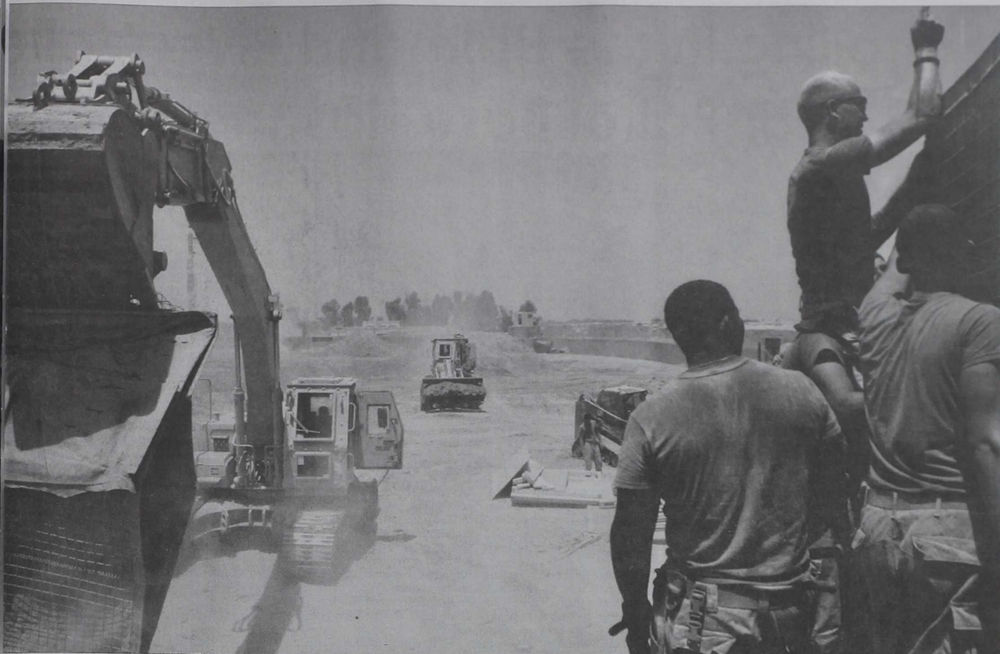
Marines with 1st Combat Engineer Battalion, put rod stabilizers in place on a Hesco barrier during construction at Patrol Base Jaker. Marines with 1st CEB, along with heavy equipment operators from Combat Logistics Battalion 8, have been working day and night building barriers and observation posts at PB Jaker, Helmand province, Afghanistan.
