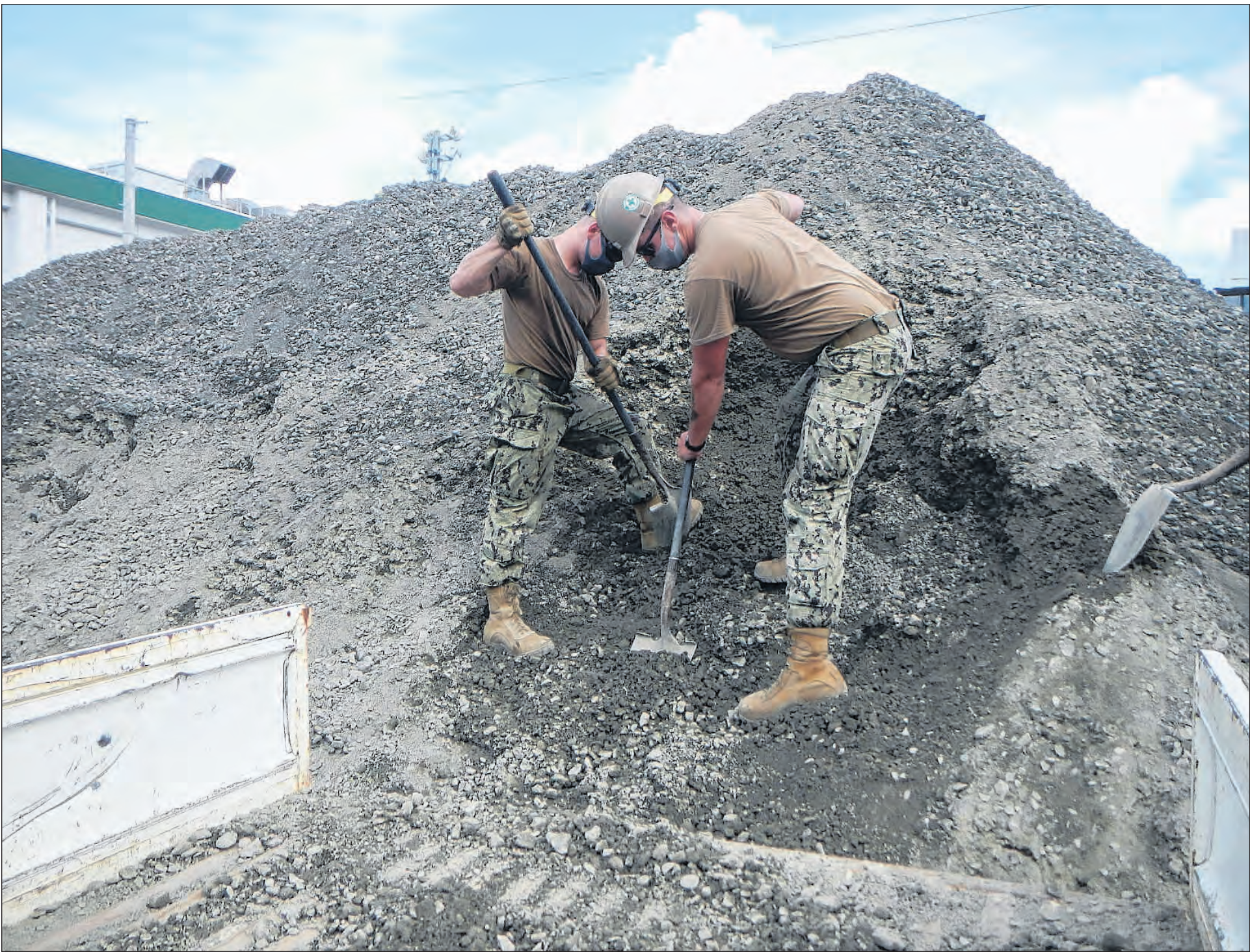
CE3 Ethan Ingle Utilitiesman Constructionman Austin Carter, from Fairgrove, Mich., and Builder Constructionman Hunter Heilmann, from Byrnes Mill, Mo., assigned to U.S. Naval Mobile Construction Battalion (NMCB) 3's Detail Sasebo, load a truck with backfilling material for footers for the construction of a pre-engineered building that will serve as a warehouse to support the storage of Naval Beach Unit 7 equipment on board Commander, Fleet Activities Sasebo, Aug. 18.
