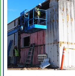
The FHL Logistics Readiness Center and several other buildings are undergoing an exterior facelift (also known as skinning) to replace the woodpecker-damaged wall. The new desert beige color blends in with other newer buildings and helps with energy efficiency. According to the installation Master Plan, buildings are updated every year to meet building requirements.
