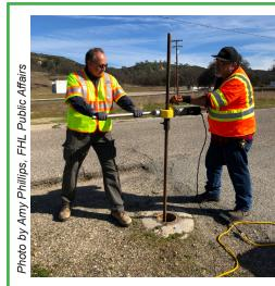
The FHL Potable Water Supply System consists of pipelines, water shut off valves, and fire hydrants installed between the 1950's and 1980's. A contractor is replacing some of the broken valves to enhance the ability of Water Operators to isolate problems and conduct repairs. Above, Dale Oviedo and Ron Garner, Utility Systems Operators exercise an underground Water Distribution System valve.
