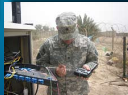
Below: Spc. Brian Robinson of the 656 Signal Co. splices fiber optic cable for the base defense operation center camera system in May. The camera system allows the BDOC to monitor the area outside of Camp Taji. Photo by Spc. Randolph Johnson
