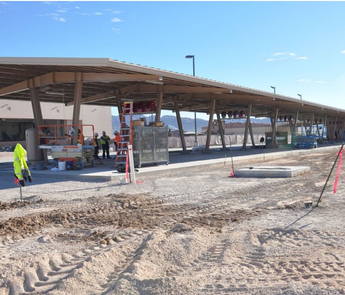
Workers at the site of the new Aviation Ground Equipment facility on Nellis AFB work on one of the exterior work bays. The Los Angeles District’s Nellis Resident Office is working on construction of the new facility which will contain interior and exterior work bays in addition to an enclosed area to power wash the equipment. (Photo by Daniel J. Calderón)
