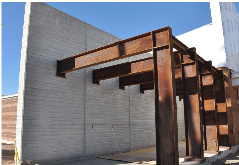
The “weathered steel” look of the framing outside the Squadron Operations Building being built by the U.S. Army Corps of Engineers Los Angeles District’s Roadrunner Resident Office at Luke Air Force is an architectural feature designed to help ease the cost of maintenance because it does not need to be repainted over and over. The building is part of a project in which the District is constructing both it and the Aerial Maintenance Unit #1 and is due for turnover to the base in December. (Daniel J. Calderón)
