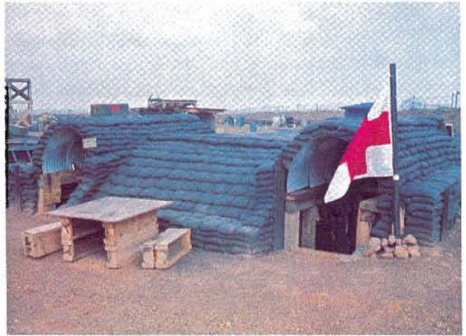
This medical bunker is typical of the interior bunkers at the fire support base. Waterproofing was provided by roofing felt, soil cement, penepime and treated sandbags.
