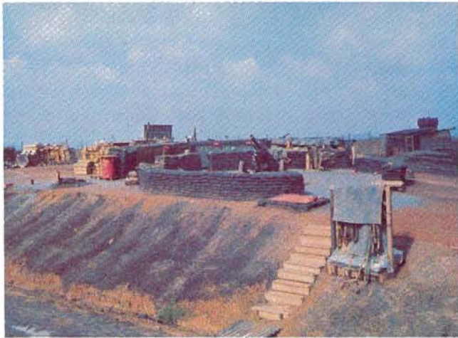
The elevated 105 artillery pad provided good stabilization and a capability for direct fire across the eight foot high firebase berm.
