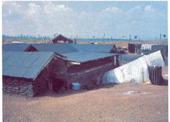
The food preparation, storage, and serving areas were also underground. The gabled roofs cover the culvert and PSP ventilation system.
