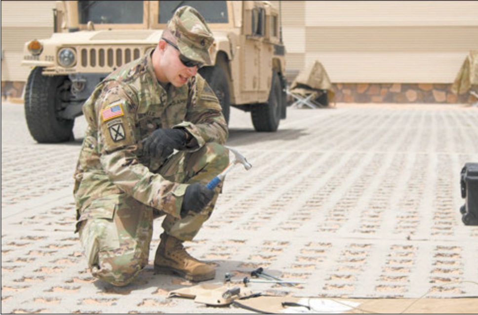
Spc. Matthew Marcellus / 1st AD Staff Sgt. Joshua Polle, a multichannel transmission systems operator-maintainer with the 1st Armored Division's G6 staff, hammers a stake to secure and anchor the Transportable Tactical Command Communications system May 2 at the Mission Training Center at Fort Bliss.
