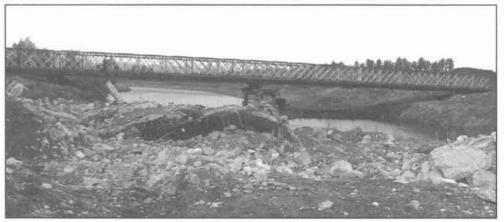
Figure 3. A bypass bridge made of DMS-65 structure elements with a continuous beam of 33 meters + 33 meters in length and access spans of 3 meters in length. The remaining parts of a destroyed bridge of 59 meters in length (Pilce town on the Nysa Klodzka River) are shown in the foreground.
