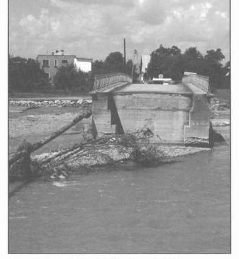
Figure 2. A washed out embankment behind a bridgehead. A 60-meter section of the access road was destroyed (Bystrzyca Dolna town - Bystrzyca River).
