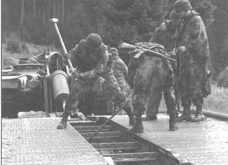
Engineers from Alpha Company, 82nd Engineer Battalion, remove a bridge near the town of Olivo, Bosnia-Herzegovina.
