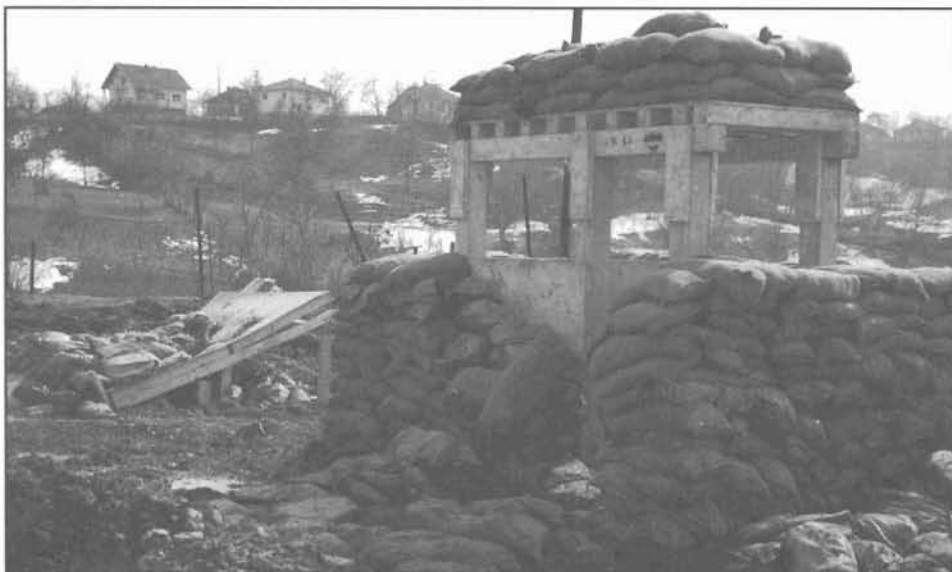
This protective bunker collapsed due to improper sandbagging.
