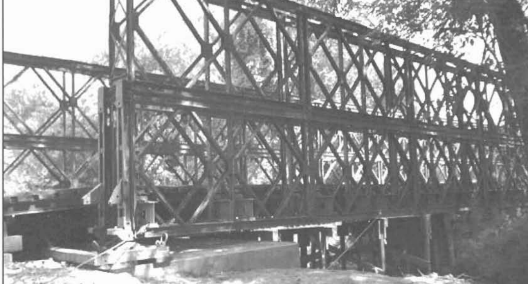
Double story MLC 70T Bailey bridge erected in June 1998 as a temporary replacement bridge at Fort Pickett, Virginia, by the 1031st Engineer Company (Panel Bridge), Virginia Army National Guard.
