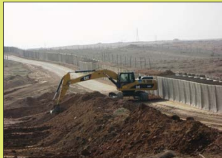
A track hoe fills Hescos along the COB Marez Perimeter in Iraq. (Photo by Sgt. 1 st Class Kelly Magleic)
