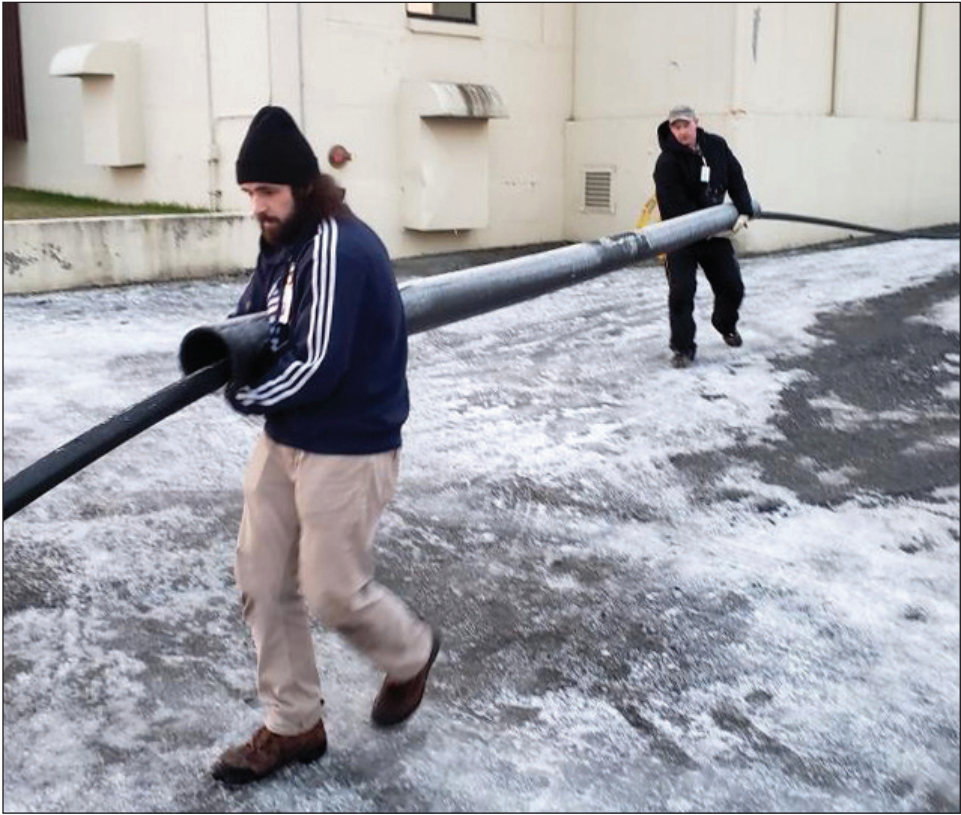
Aaron Bryant and Rick Gill, 773d CES utilities operators, assemble a 300-foot section of insulated pipe at Joint Base Elmendorf-Richardson Dec. 1, after an earthquake broke the water main. (Courtesy photo)
