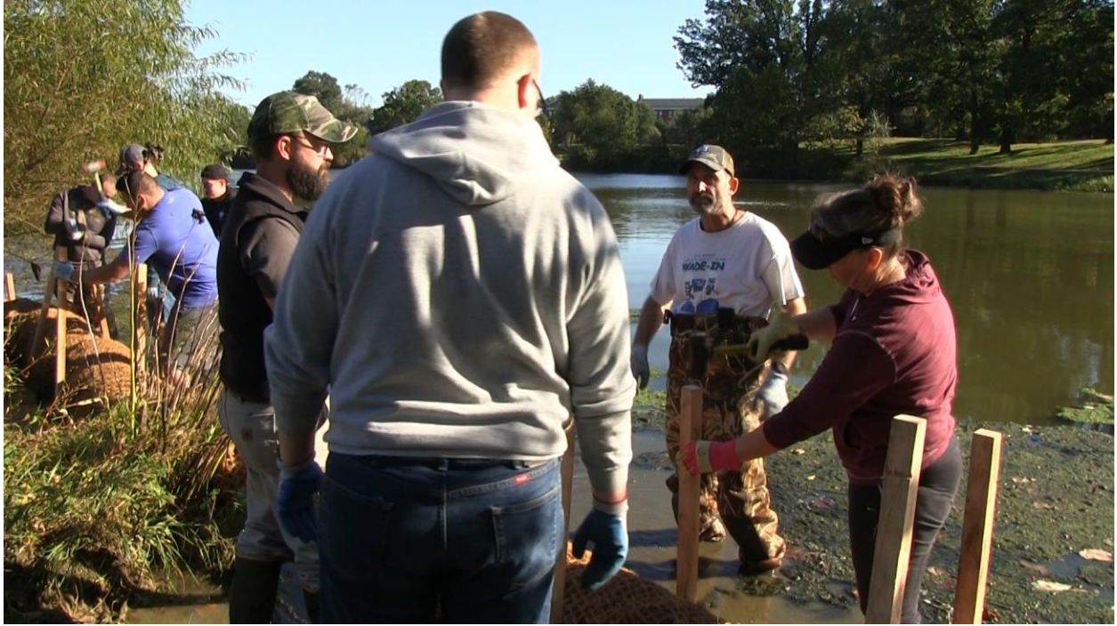
Deborah Patterson and Mitch Keiler of the DPW Environmental Division pound 4-foot stakes into the Burba Lake bed. The stakes will keep in place the bio-log.
