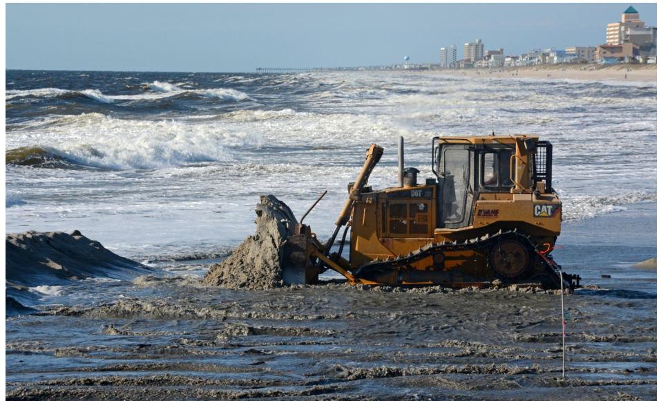
A bulldozer moves dredged material on the north end of Carolina Beach.
