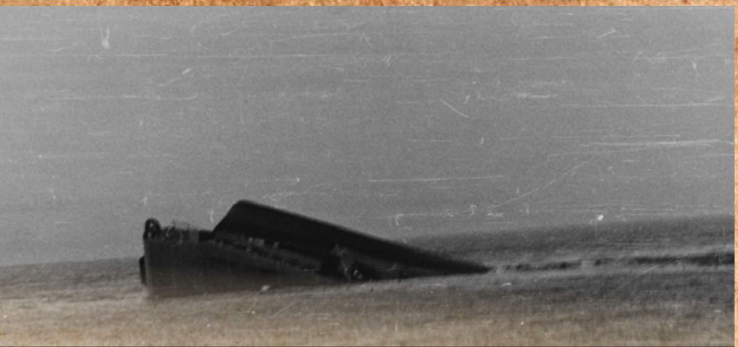
USS Yorktown (CV-5) sinking, just after dawn on 7 June 1942, as seen from an accompanying destroyer. The ship has capsized to port, exposing the turn of her starboard bilge, and is settling rapidly by the stern. This view looks over the ship's upper starboard structure, with her forefoot and front edge of the flight deck in the left center. Note froth at right from escaping air. U.S. Naval History and Heritage Command Photograph.
