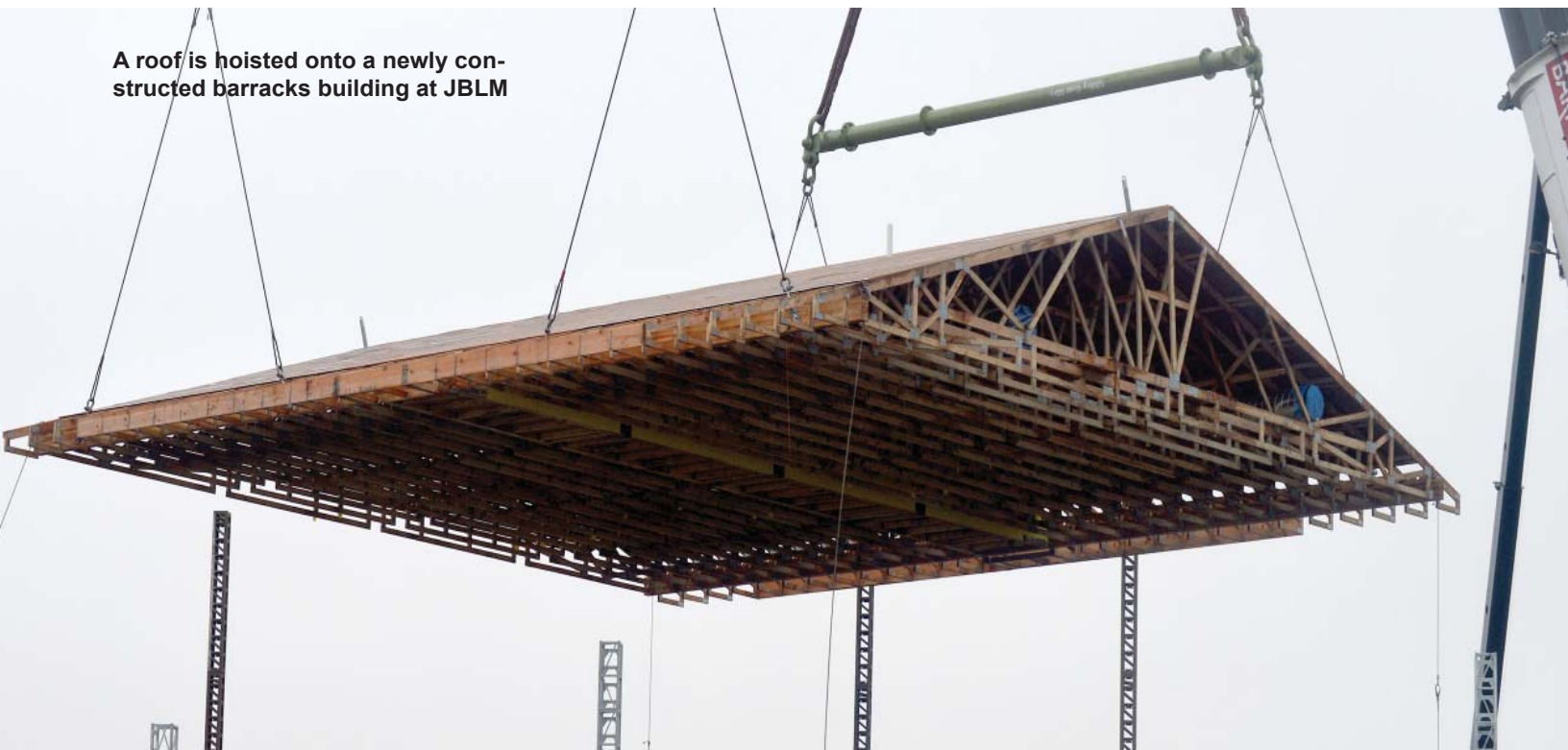
A completed roof section sits ready to be hoisted onto a barracks building.
