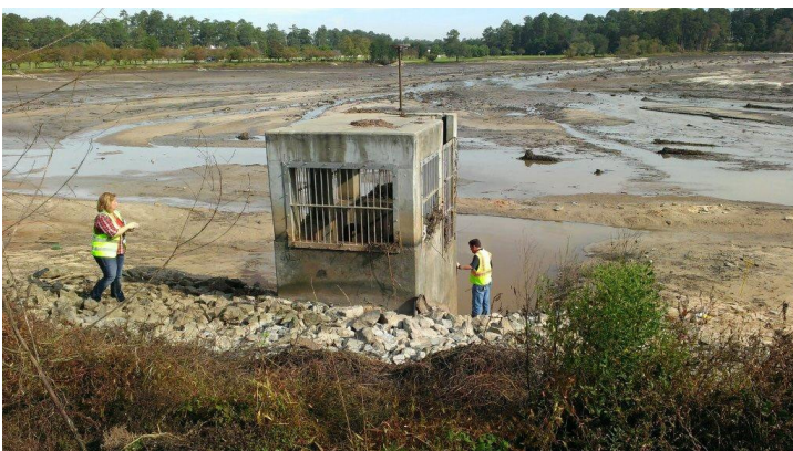
Shannon Geoly and Mitch Hall inspect an intake valve structure at the Semmes Lake Dam site.
