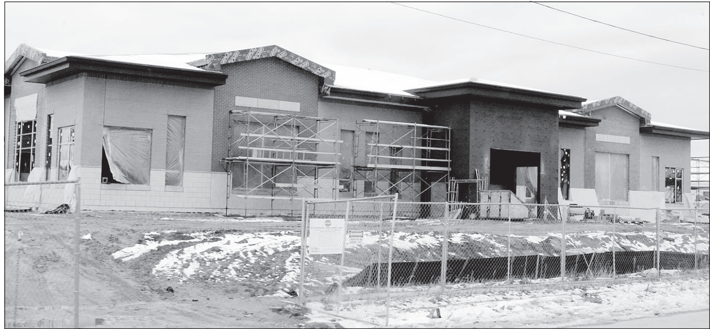
Construction continues on the new annual training/mobilization dining facility at Fort McCoy. The $7.7 million project is scheduled to be completed in June.
