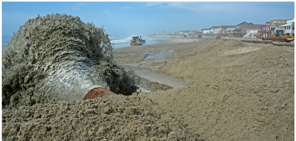
Dredged material spews on Ocean Isle Beach as a bulldozer prepares to sculpt it to the proper elevation. (USACE photos by Hank Heusinkveld)
