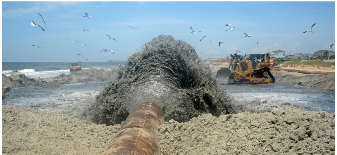
Dredged material from Smith Island Channel spews onto Caswell Beach as a bulldozer moves material around to bring it to the proper elevation to help reduce risks to oceanfront property. (USACE photo by Hank Heusinkveld)
