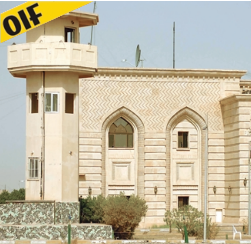
The Hospitality Palace, once Saddam Hussein's smallest palace, is now the headquarters building for the 4th Iraqi Army Division, located on Forward Operating Base (FOB) Dagger near the village of Saddam's birth.
