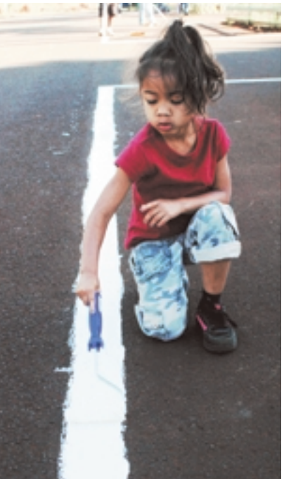
Content as can be, Skyley Goodman, 5, daughter of Sgt. 1st Class Jeffrey Goodman, platoon sergeant, 66th Engineers, helps restripe the parking lot entrance to Helemano.
