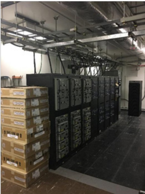
The finished product included nine new racks, 24 new radios and thousands of feet of new cable all installed by the EI team.
