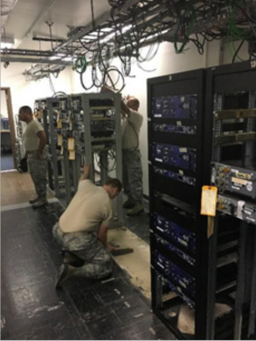
Members of the 243rd EIS work to remove old equipment and racks making space for the new CM-300 radios and associated infrastructure.
