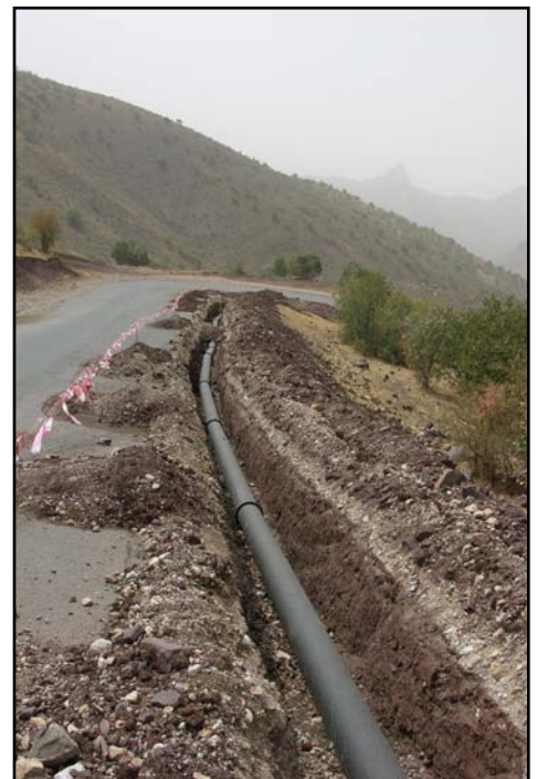
Five miles of pipe delivers mountain-top spring water to the town of Choman below and its two neighboring villages, where it connects to an existing water network. Approximately 40,000 people will go from two hours of water every three days, to three or four hours of water every day when the Irbil projects are completed.
