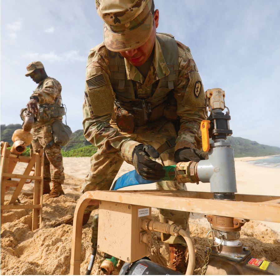
Photo by Sgt. Ian Ives, 25th Sustainment Brigade Public Affairs, 25th Infantry Division SCHOFIELD BARRACKS — Soldiers from the 209th Aviation Support Battalion, 25th Combat Avn. Brigade, 25th Infantry Division, assemble a water pump, Feb. 27, near Dillingham Airfield, prior to beginning the water purification process. The Support Operations cell, 25th Sustainment Bde., 25th ID, oversaw the 209th ASB training on the Tactical Water Purification System, which will help build water purification proficiency in the Pacific theater.
