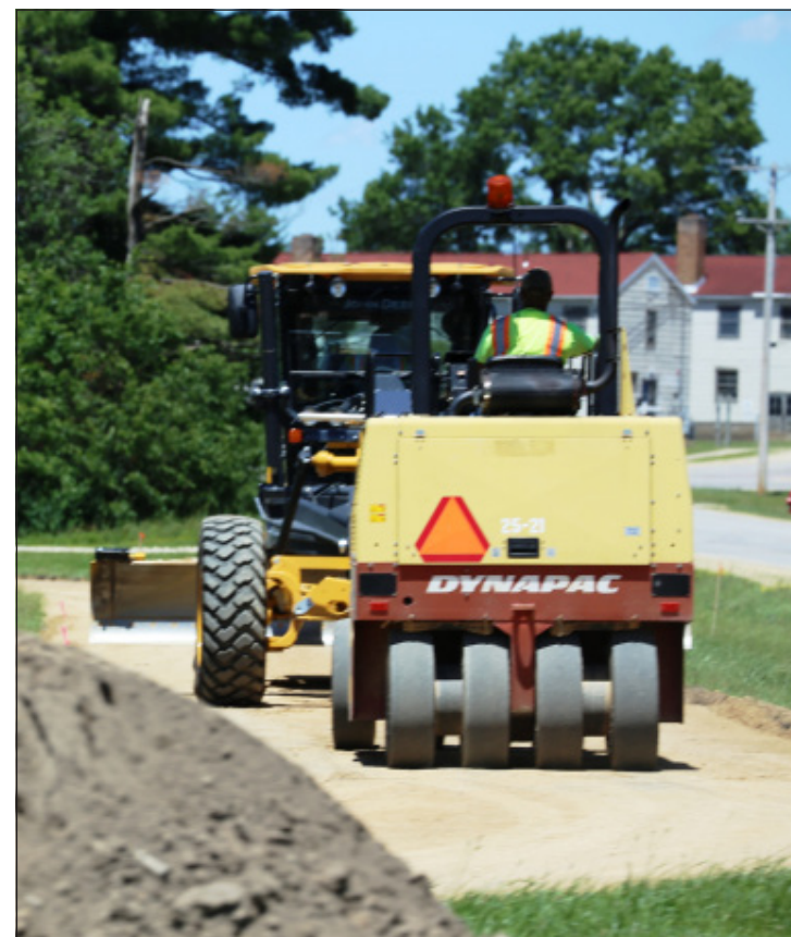
Workers with contractor Mathy Construction of La Crosse, Wis., work on resurfacing the running track June 14 at the Fort McCoy Physical Fitness Training Site.
