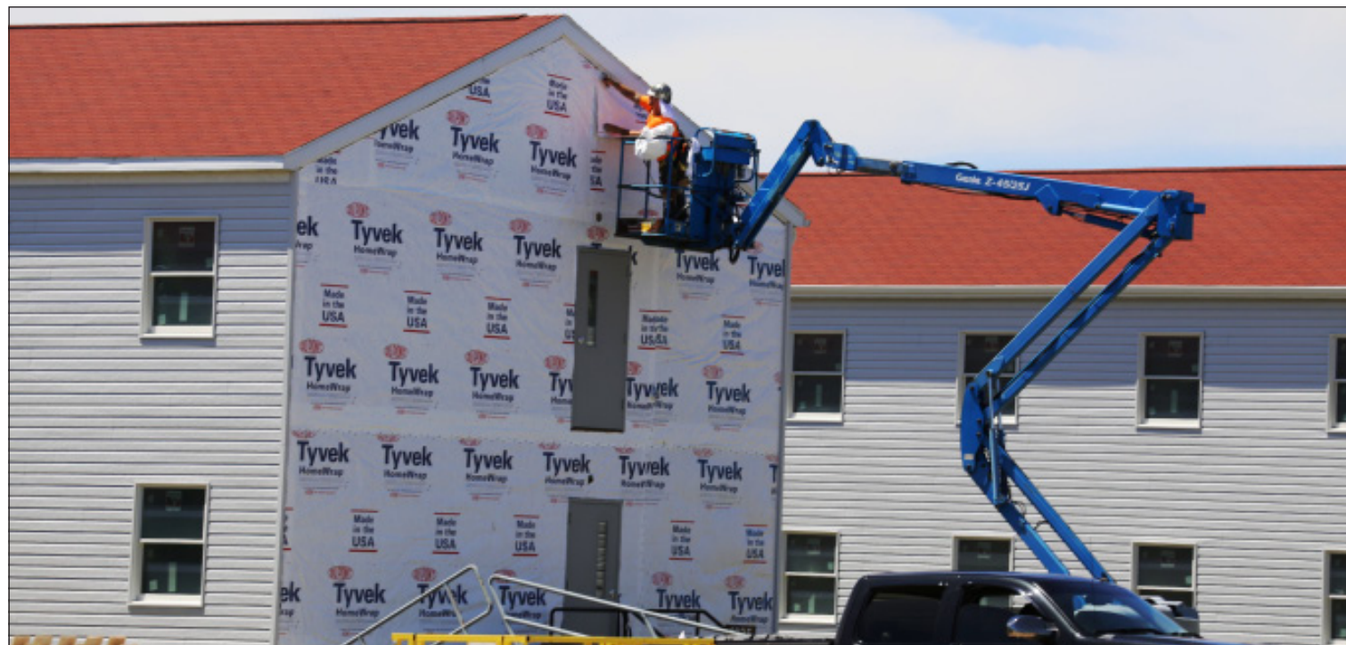
A worker with contractor Nuvo Construction of Milwaukee works on a barracks building in the 1900 block June 15 on the cantonment area at Fort McCoy.
