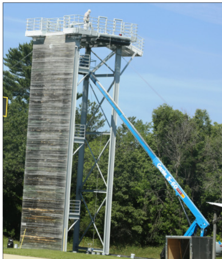
A worker with contractor Platt Construction of Tomah, Wis., works on the rappel tower June 27 on the cantonment area.
